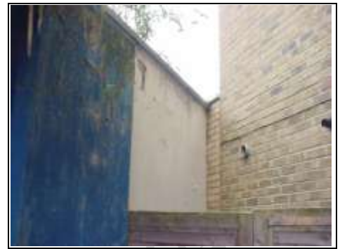
Close up of top of rear right hand side of wall
