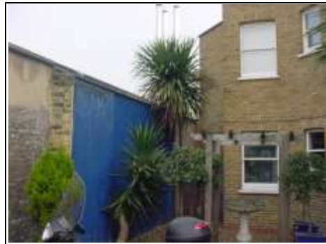
Rear right hand side of wall
