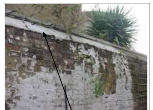
Concrete capping just below coping stone
