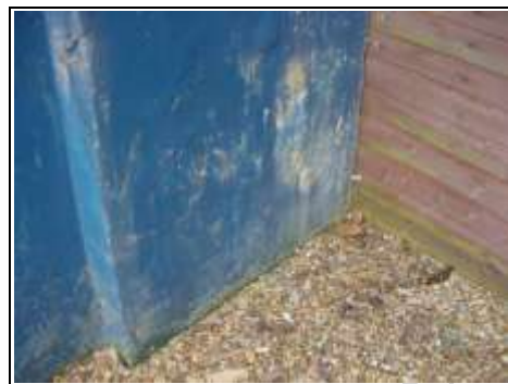
Base of rear right hand wall
