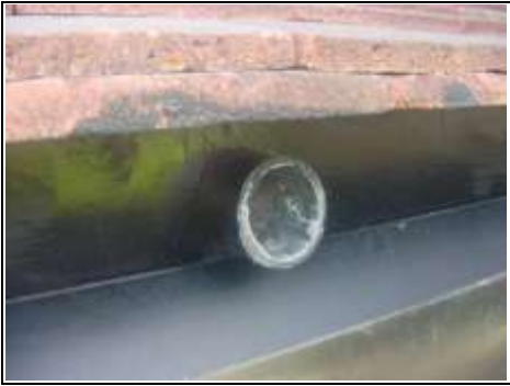
Poor gutter detailing
