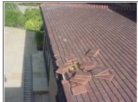
Roof opened up to expose the GRP layer below
