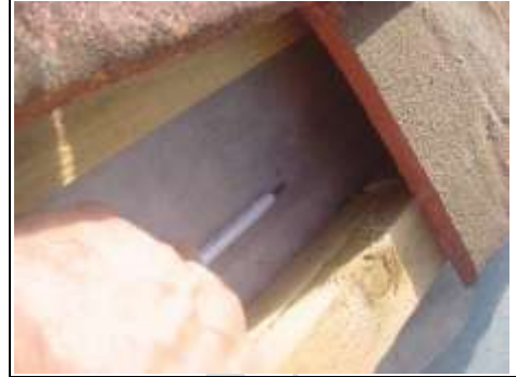
Return on GRP to pen which is not high enough
